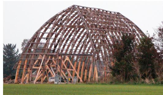
The curved rafters are formed of thin layers of timber bolted together.
