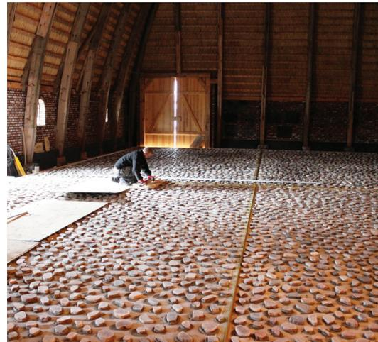
Large pebbles were laid by hand and bonded with mortar to the mesh sheet.
