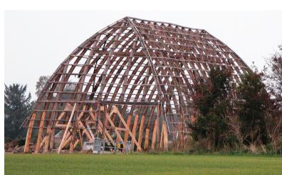
The curved rafters are formed of thin layers of timber bolted together.
